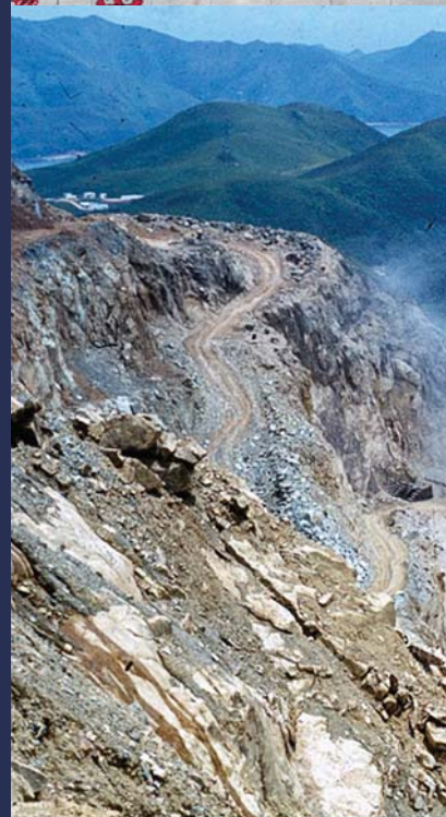
Granite quarry (at Anderson Road), photographed about 1977
