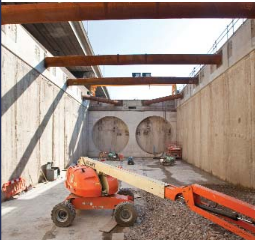
Ready for the Tunnel Boring Machine – the Royal Oak portal, west of Paddington awaits the arrival of 'Phyllis'
