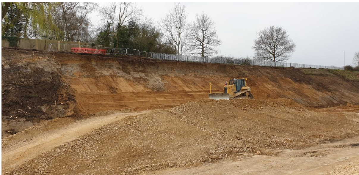
Figure 1 - Glacial fluvial deposits over Oxford Clay within a cutting slope at Winslow
