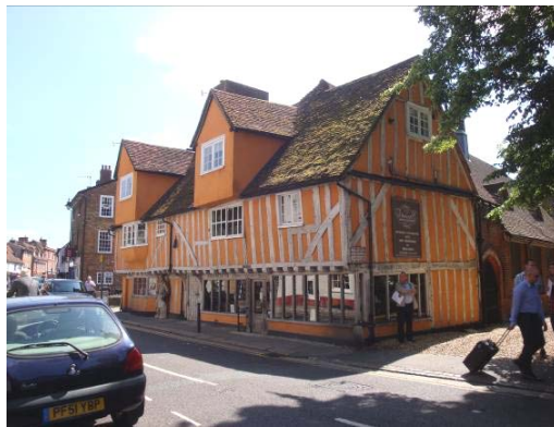
Former Verger's House, oldest residential building in Hertford
