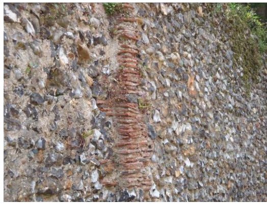
Roman tiles in curtain wall, Hertford Castle
