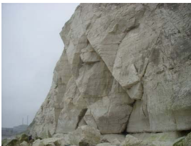
Holywell Nodular Chalk Formation – inclined conjugate fractures
