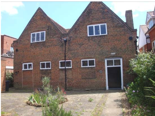
Grade 2 listed Quaker meeting house, Railway Street
