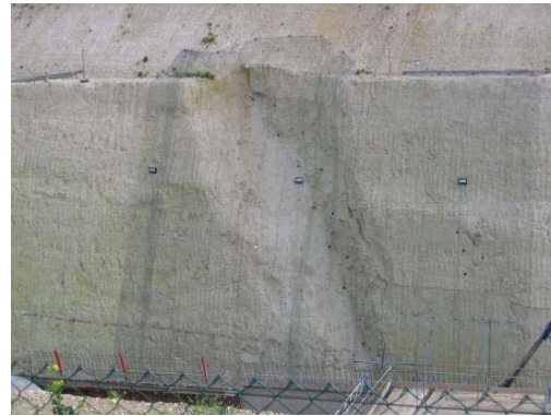
Fault across Southerham Marl, Baldock by-pass tunnel
