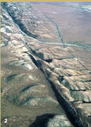
1 San Andreas fault close to Olema, San Francisco, USA, 1906. US Geological Survey, Department of the Interior/USGS photo by G K Gilbert
