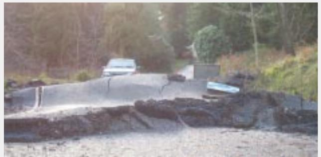
*Pictured: Damage to a road caused by the Leith Hill landslip (Surrey), which was reactivated by heavy rainfall in December 2000. Photo: Mike Stephen.*
