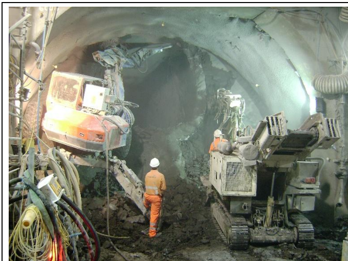
Simultaneous excavation of an enlargement and breakout of a pilot tunnel at King's Cross, 2007.
