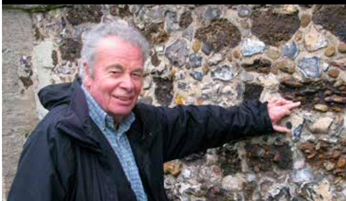
John Potter points out ferruginous gravel blocks from the Taplow Gravels in the wall of St Mary's Ripley, Surrey. Photo: Ted Nield, 2012
