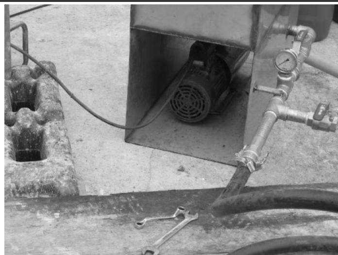
An experimental use of hydrogen peroxide in water well rehabilitation
