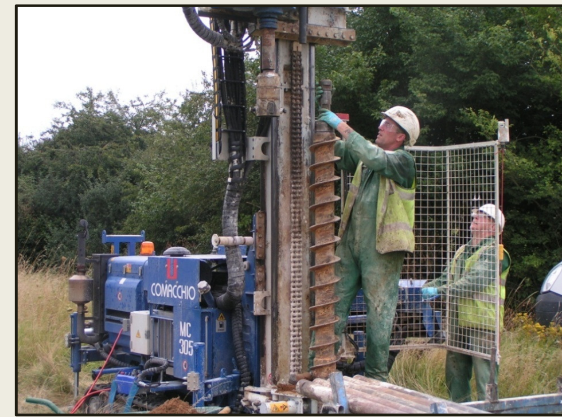
Six boreholes drilled to 18 m depth (COMACCHIO MC305 Hollow Stem Auger Rig)
