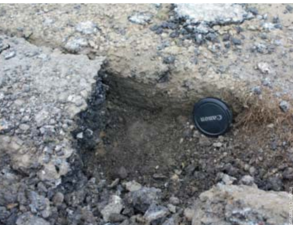
Thickness of farmacadam in-situ prior to re-surfacing treatment, unclassified road Nr Grantham
