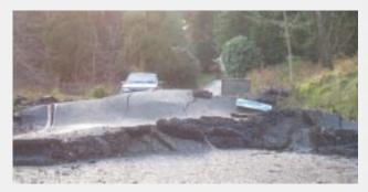
Pictured: Damage to a road caused by the Leith Hill landslip (Surrey), which was reactivated by heavy rainfall in December 2000. Photo: Mike Stephen.
