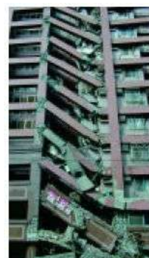
Damage caused by the Taiwan Earthquake. Photo Mike Ellis, courtesy Centre for Earthquake Research & Information, University of Memphis.
